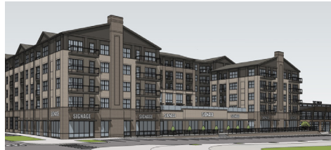
UNION SQUARE A 80,400 SF mixed-use building near Grand Junction Plaza.
